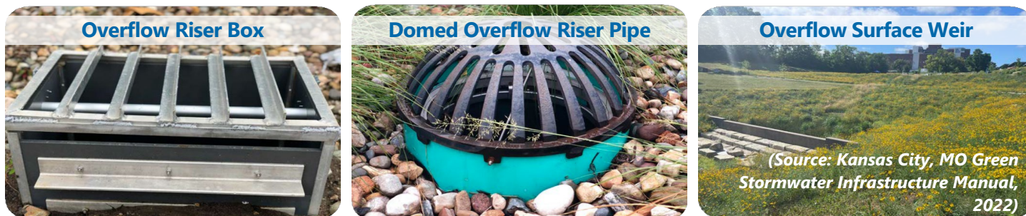
Figure 7.18-1 Typical Overflow Controls for Tier 1 and Tier 2 SCMs
