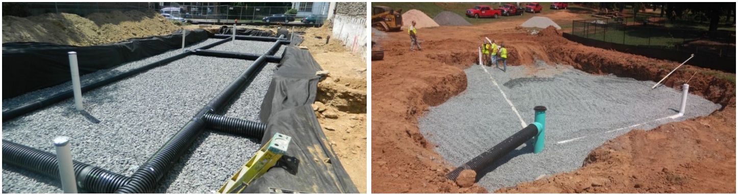
Left: SCM installation with HDPE underdrain pipe and capped PVC observation wells (Source: Philadelphia Water Department); Right: A bioretention area under construction in Salem, NC. Note the upturned elbow underdrain and capped cleanouts (Source: Hazen and Sawyer)
