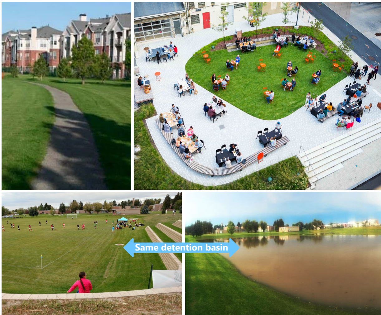
Figure 4-20 Examples of “Use of Natural Features and Preserved Areas” LID Design Practices
