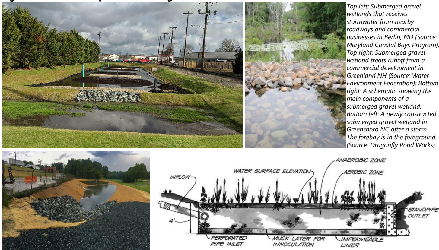
Figure 7.11-1 Examples of Submerged Gravel Wetlands
