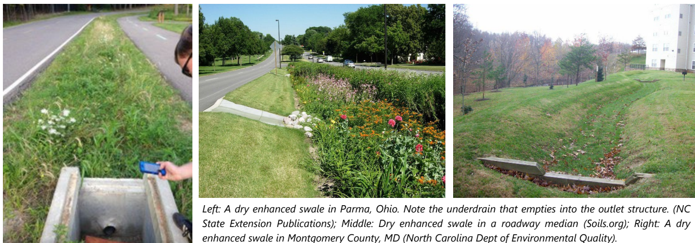
Figure 7.4-1 Examples of Dry Enhanced Swale Applications
