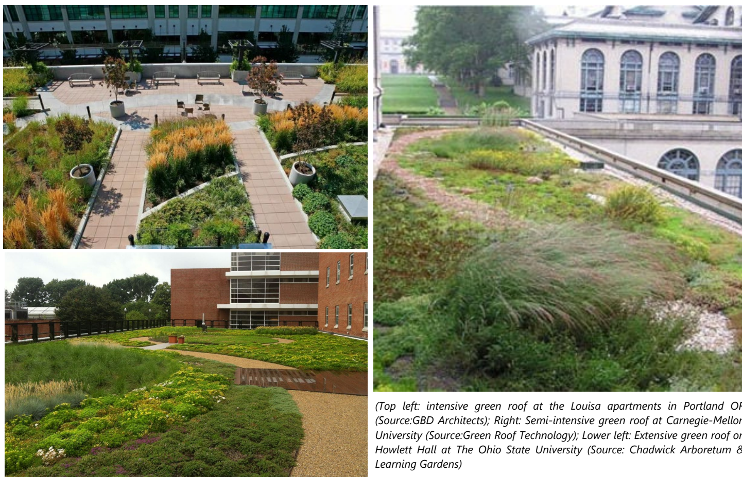
Figure 7.5-2 Examples of Intensive and Extensive Green Roofs
