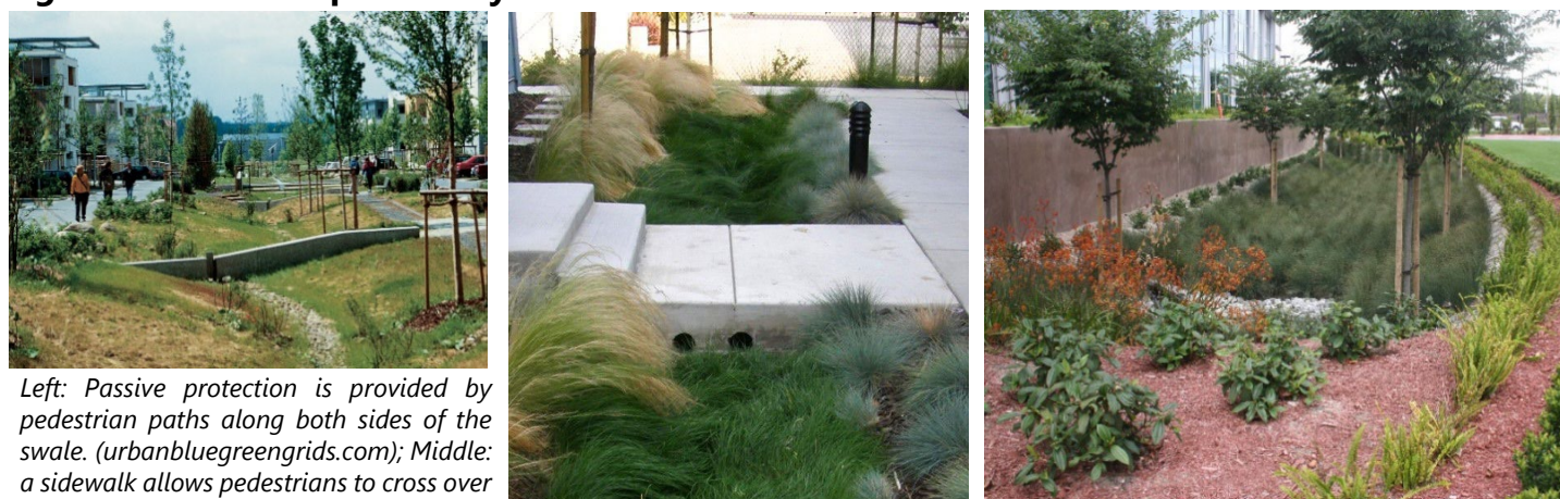
Figure 7.4-3 Examples of Dry Enhanced Swale Protection Measures
