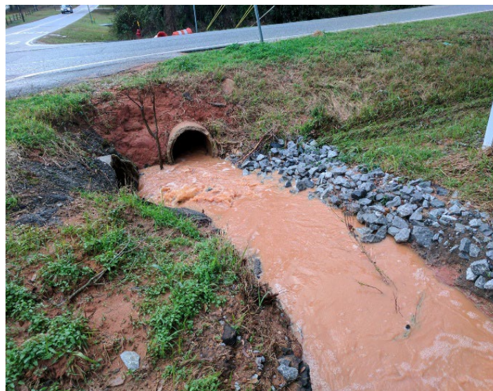
Figure 2-6 Sediment Laden Stormwater
