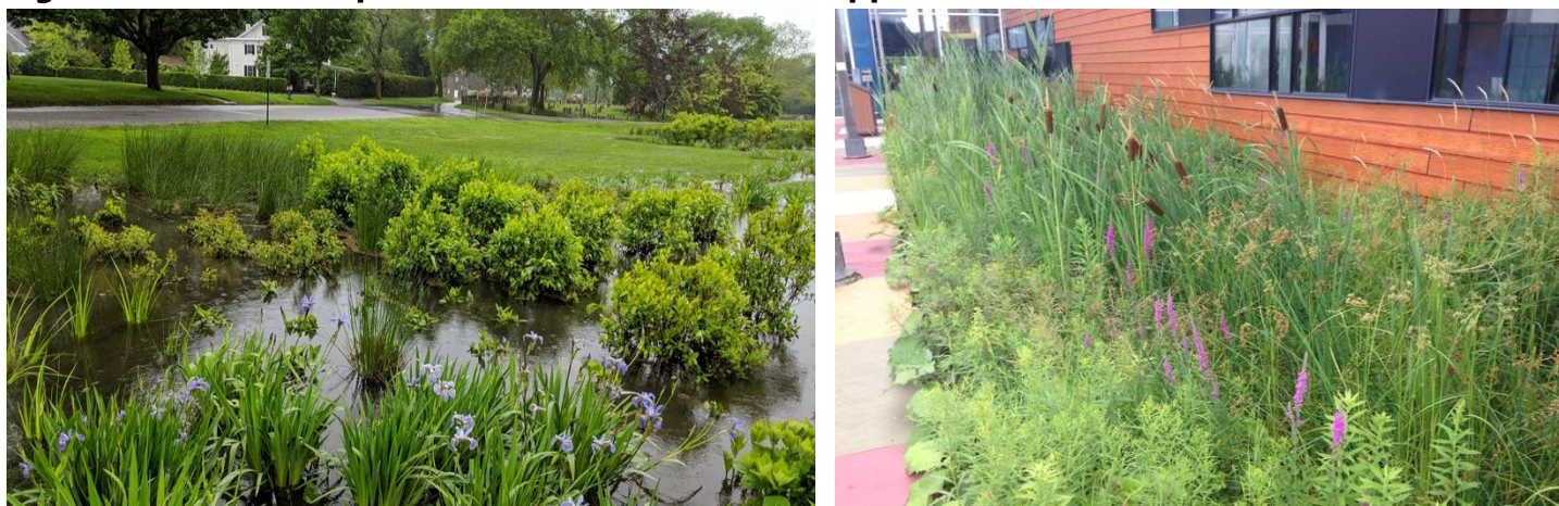
Left: A wet enhanced swale receives drainage from a roadway in East Hampton, NY. (Source: tomtwomeyseries.org); Right: A wet swale in Montreal, Canada (Source: NC State Extension Publication AG-588-26, Feb. 10, 2020)
