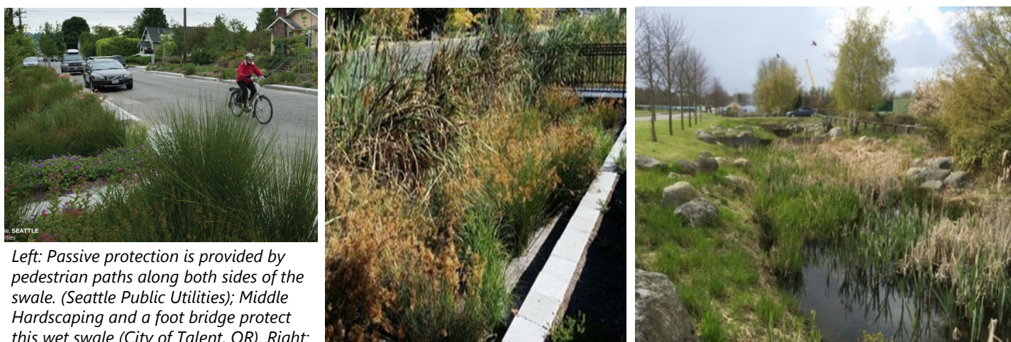
Figure 7.14-4 Examples of Wet Enhanced Swale Protection Measures
