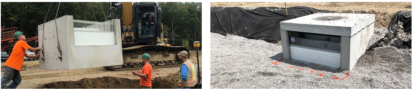
Figure 7.16-14 Installation of a Proprietary Treatment Device (Source: ACF Environmental/PRETX system)
