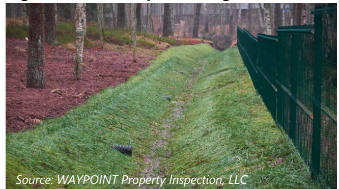
Figure 4-22 Examples of Vegetated Swales
