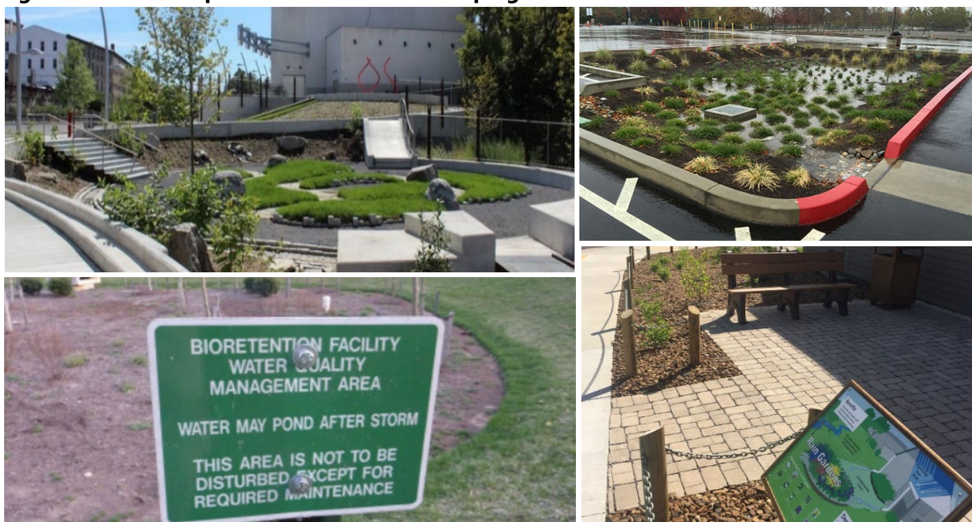
Top Left: Pathways along and through a bioretention area guide pedestrians to appropriate places to walk (City of Philadelphia, PA Water Dept); Top Right: Concrete curbing around a parking lot bioretention area keeps vehicles and people out while allowing stormwater in (Sacramento State University); Bottom Right: Decorative fencing, benches, and signage all help protect this bioretention area (City of Oak Ridge, TN); Bottom left: A sign indicating the presence of an SCM and prohibiting disturbance. (source unknown).
