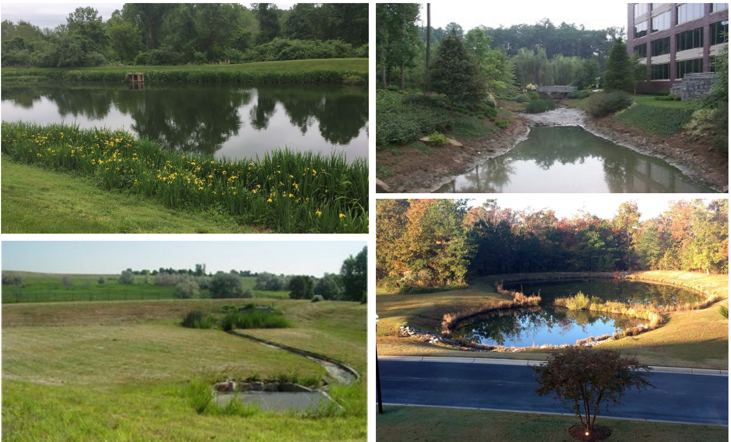
Top left: A wet pond located at the Risteau at Rockland in Baltimore County, MD; Top right: A wet ED pond (location and source unknown); Bottom right: A multiple pond system in Brunswick County, NC (Source: NC State Extension); Bottom left: A micropool ED pond at Grant Ranch in Denver, CO (Source: Mile High Flood District)
