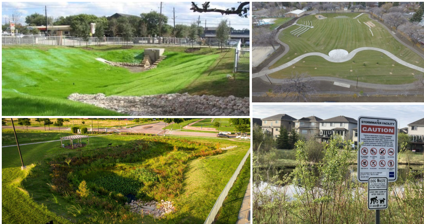
Top Left: Fencing can be installed around a basin's permitter (City of White House, TN); Top Right: Some basins are designed for dual purposes. This basin is used as recreational areas. (Sacramento State University); Bottom Right: Safety signage installed at a detention basin in Edmonton, Canada (Jolyn Hall, Schmidt Realty Group, inc. ); Bottom Left: Landscaping can deter people and vehicles from entering a detention basin in Houston, TX (photo: Bryan Malloch).
