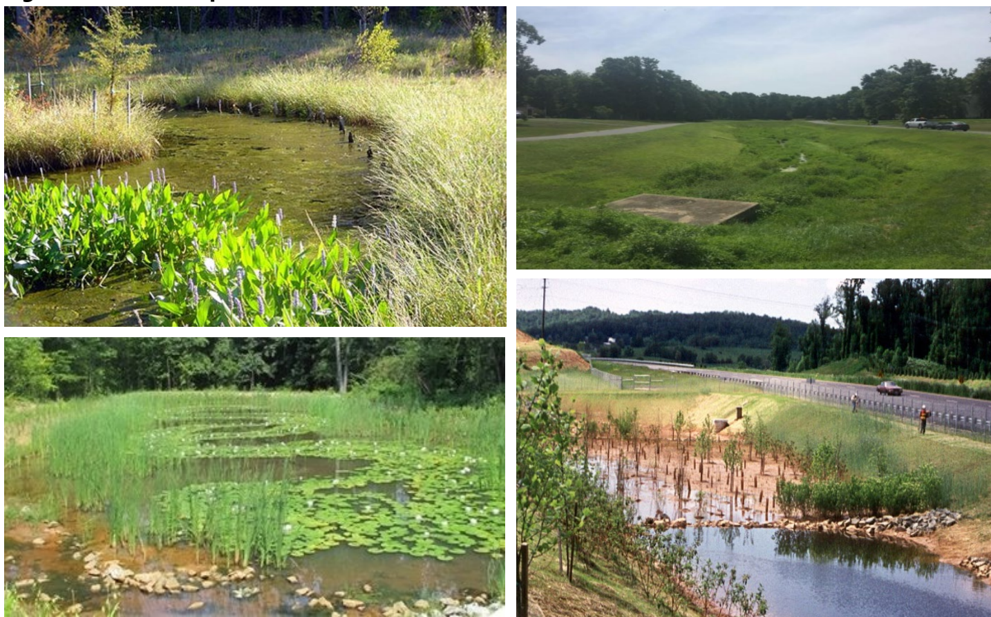
Top left: Shallow wetland (Maryland Department of Transportation); Top right: Extended detention shallow wetland (Maryland Department of Environment); Bottom right: Basin/wetland system (Connecticut Stormwater Quality Manual); Bottom left: Pocket wetland (Athens-Clarke County, GA)
