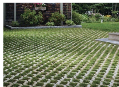
Figure 7.8-1b Concrete Grid Pavers
