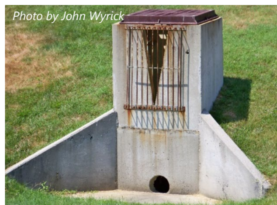
Figure 7.3-1 Example of a Multi-Stage Outlet Structure
