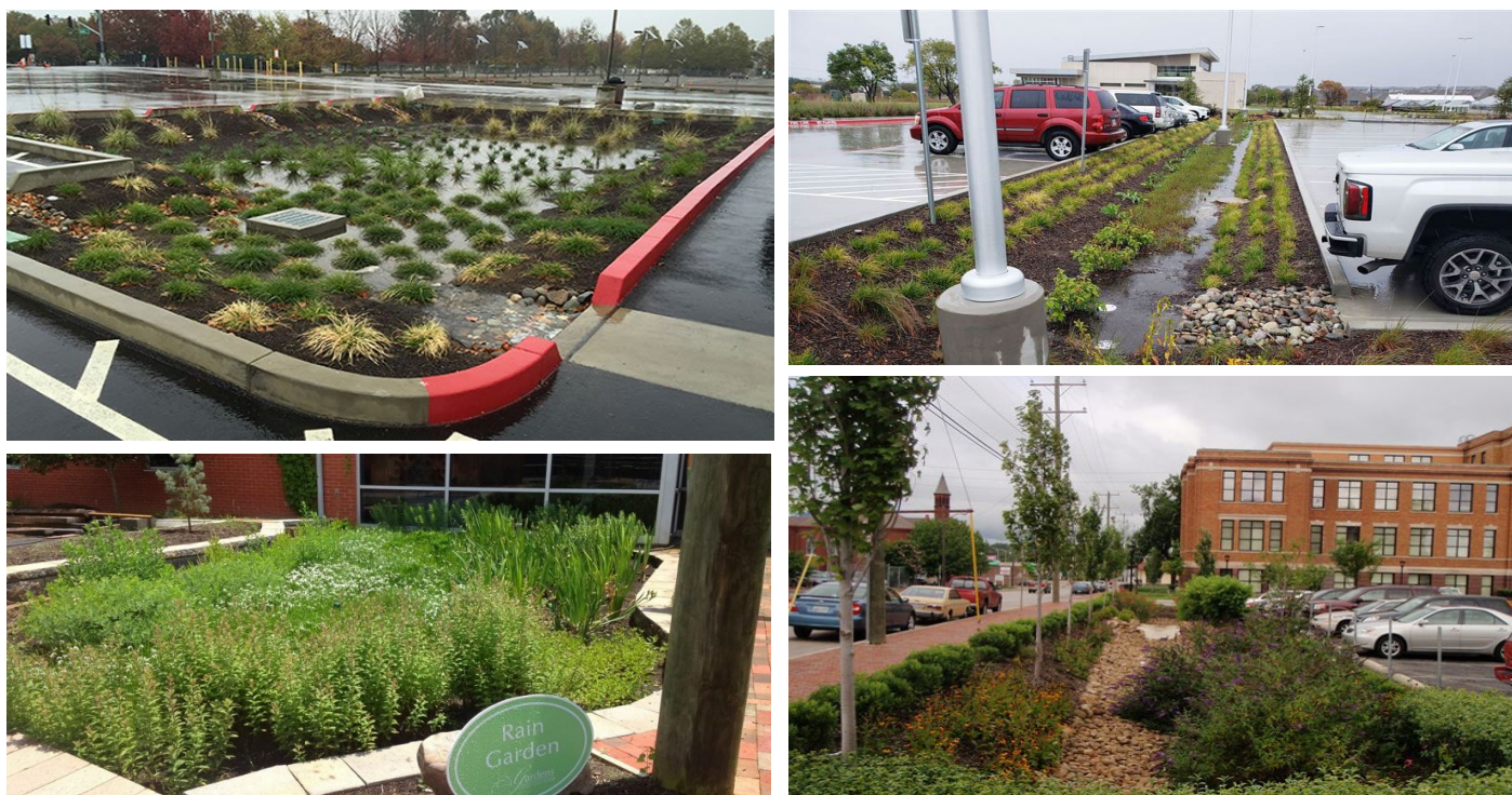
Figure 7.1-1 Examples of Bioretention Area Applications
