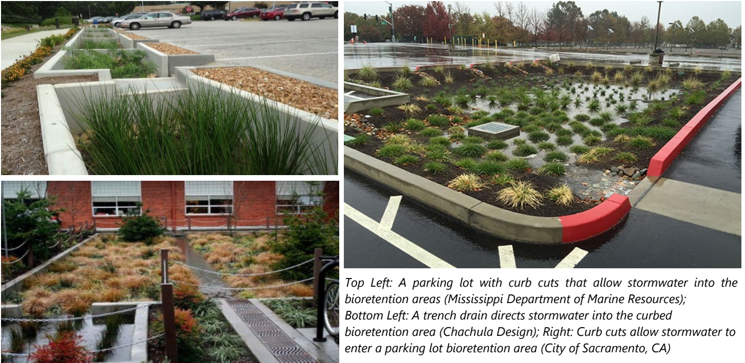
Figure 7.16-2 Examples of Different Curb Openings
