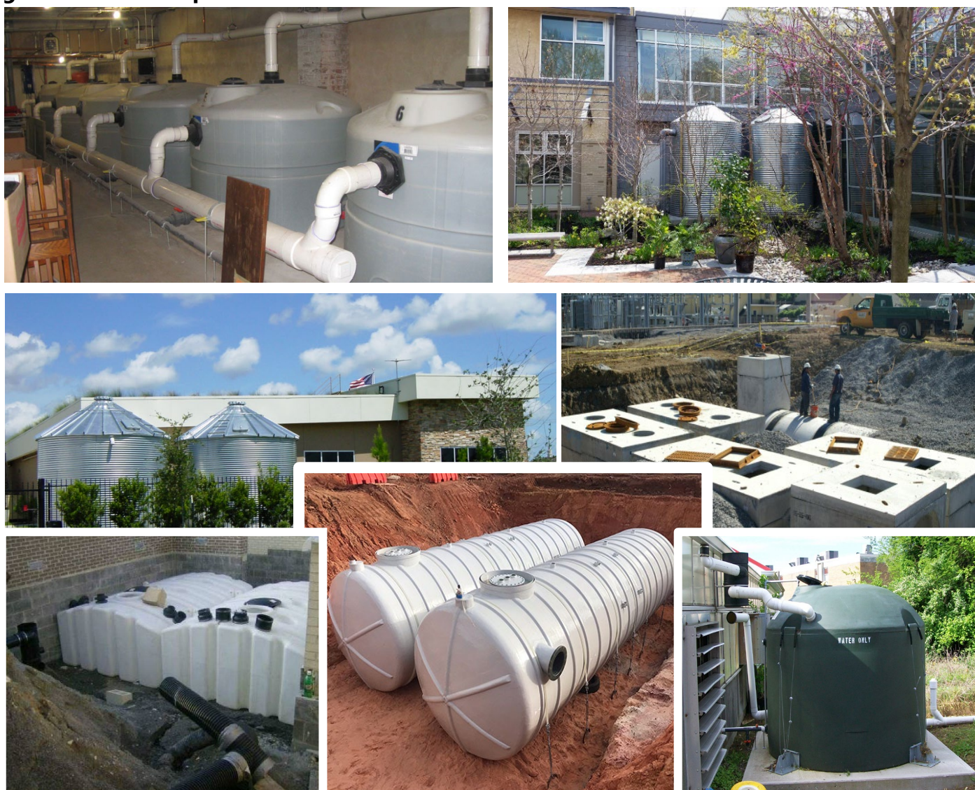
Figure 7.2-1 Examples of Surface and Subsurface Cisterns
