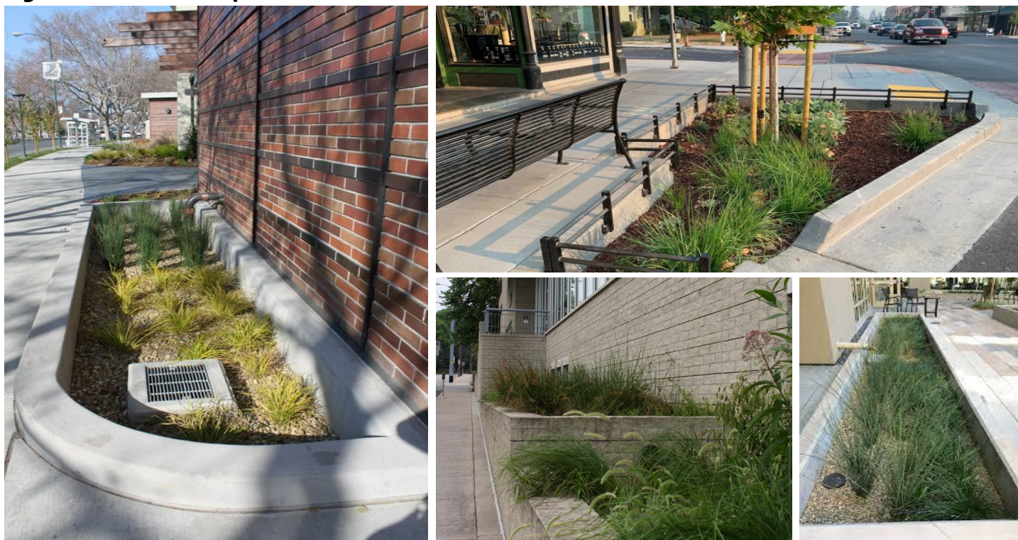
Left: An urban bioretention serves receives roof runoff through a downspout and serves as a decorative planter box; Upper Right: Urban bioretention areas manages runoff from the sidewalk and street in the City of Ukiah, CA (Source: Russian River Watershed Association); Lower middle: Urban bioretention boxes at the Tennessee Association of Realtors in Nashville TN (Metro Water Services); Lower Right: An urban bioretention area receives stormwater from the downspout of the adjacent building
