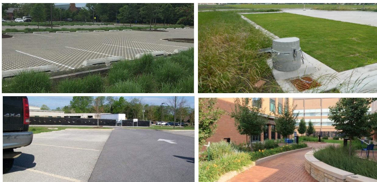
Figure 7.8-2 Examples of Permeable Pavement System Applications
