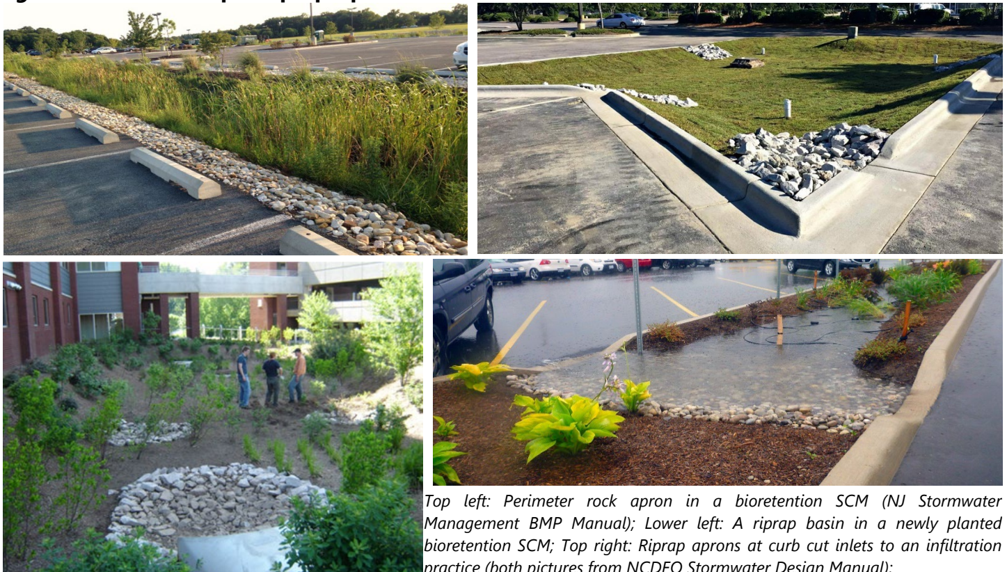
Figure 7.16-5 Example Riprap Aprons
