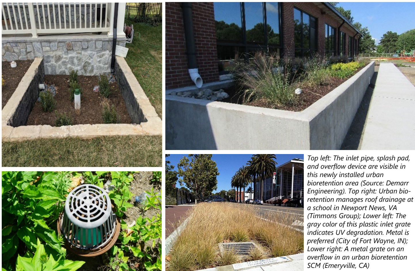
Figure 7.13-5 Examples of Inflow and Overflow Structures
