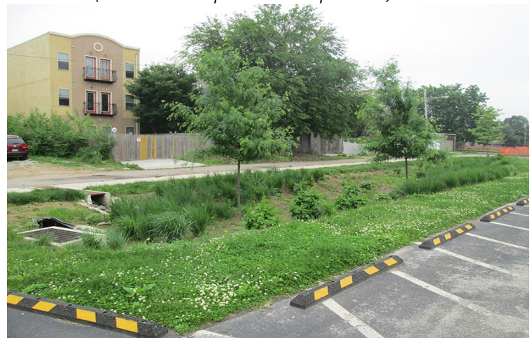
Figure 7.16-10 Example of Grass Filter Strip
