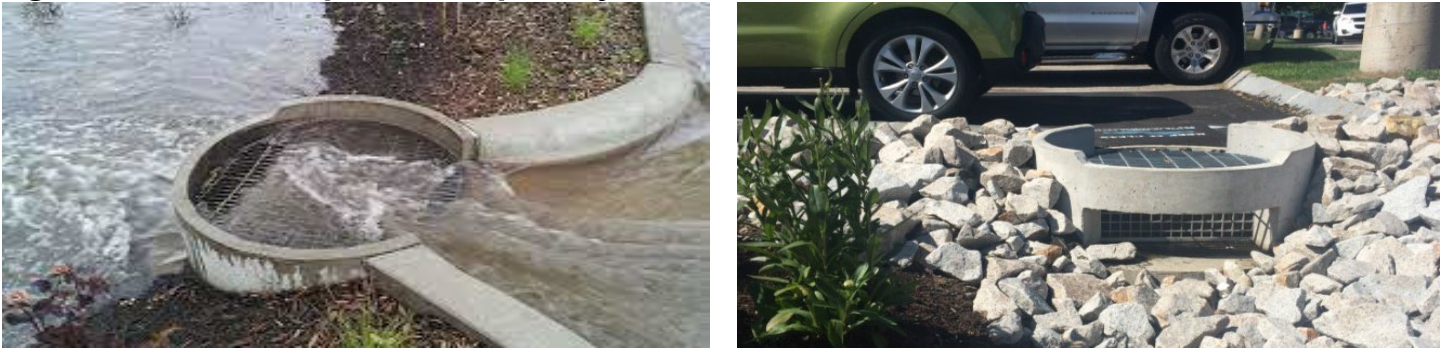
Figure 7.16-13 Example of a Proprietary Pretreatment Device (Source: Rain Guardian)
