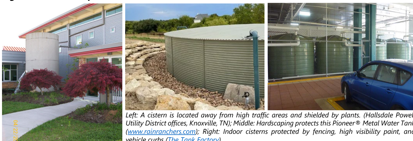
Figure 7.2-4 Examples of Cistern Protection
