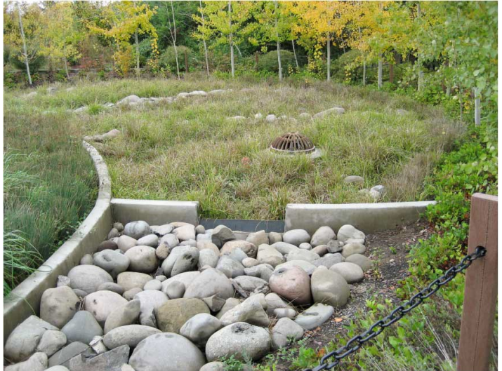
A bioretention area’s forebay (also rock basin or rip rap basin) is shown in the foreground. Picture source: Water Conservation Technologies
